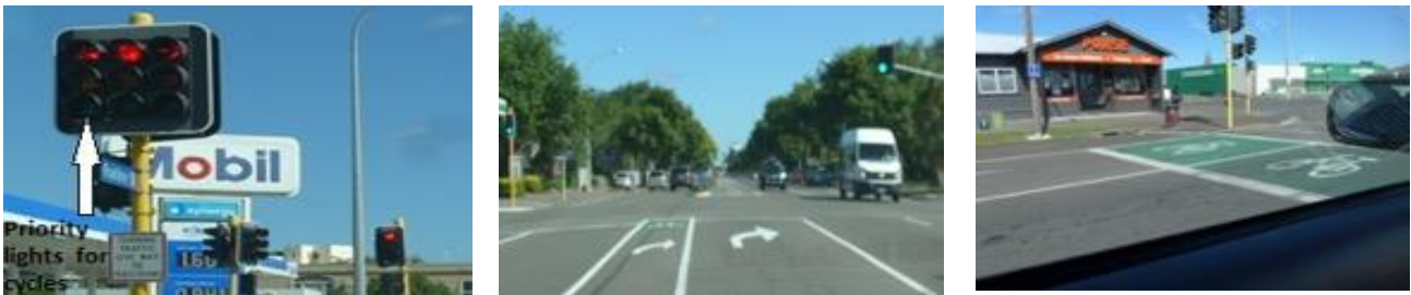
Figure 6.9: Examples of prioritising bicycles at intersections, including priority traffic lights and intersection
