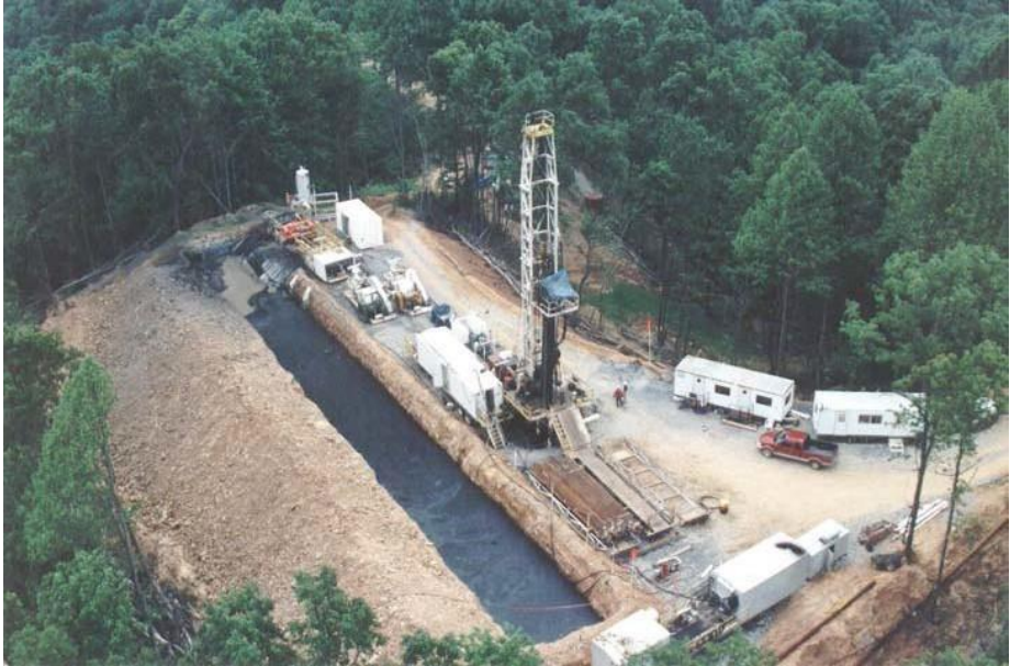
Figure 3.19 CDX Drilling Rig on Location in Central Appalachian Basin
