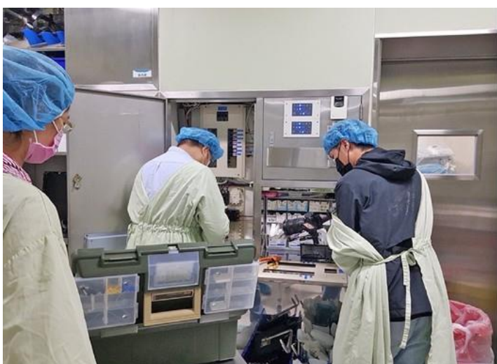
Figure 4. Installation of environmental control box in operating rooms
