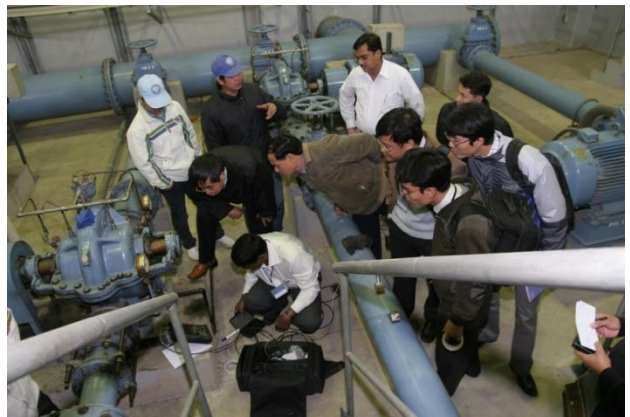
Water Flow Measurement
