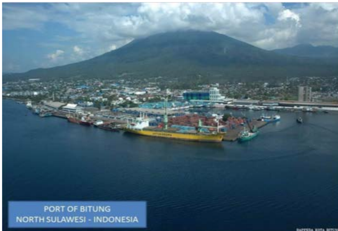
Figure 2: Port Facilities at Bitung (Credit: Bitung City)
