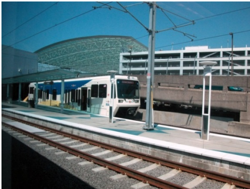
Image 48. MAX Red Line Tram Station
