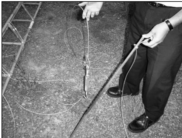
Photo 13-1: Guy Wires and Turnbuckle
