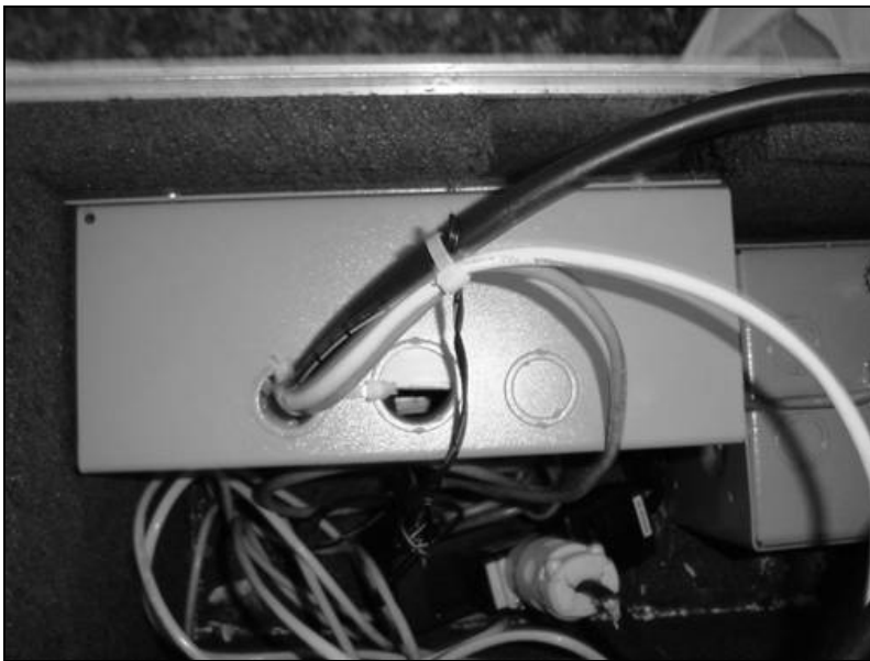
Photo 12-3: Details of AP Connections inside Enclosure
