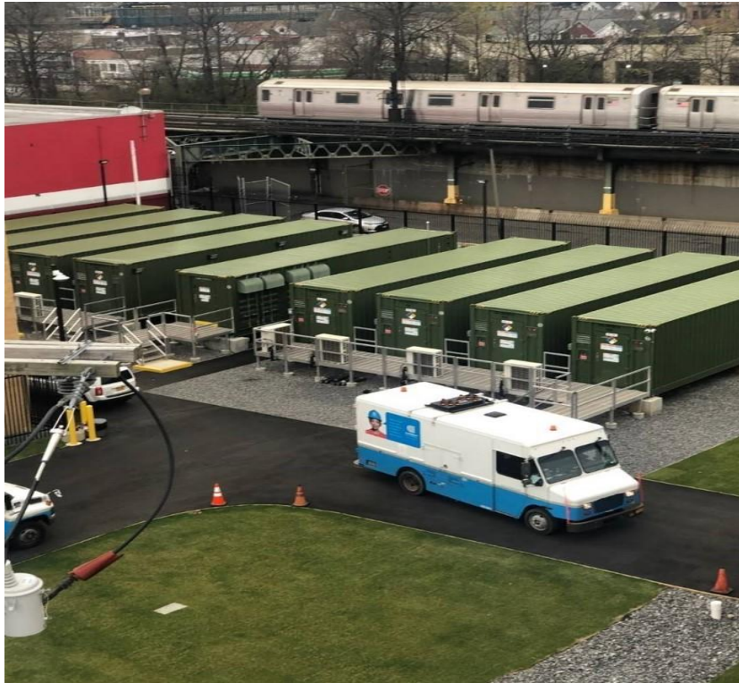
Figure 6-7 Con Edison's 2MW/11MWh Storage System in Ozone Park
