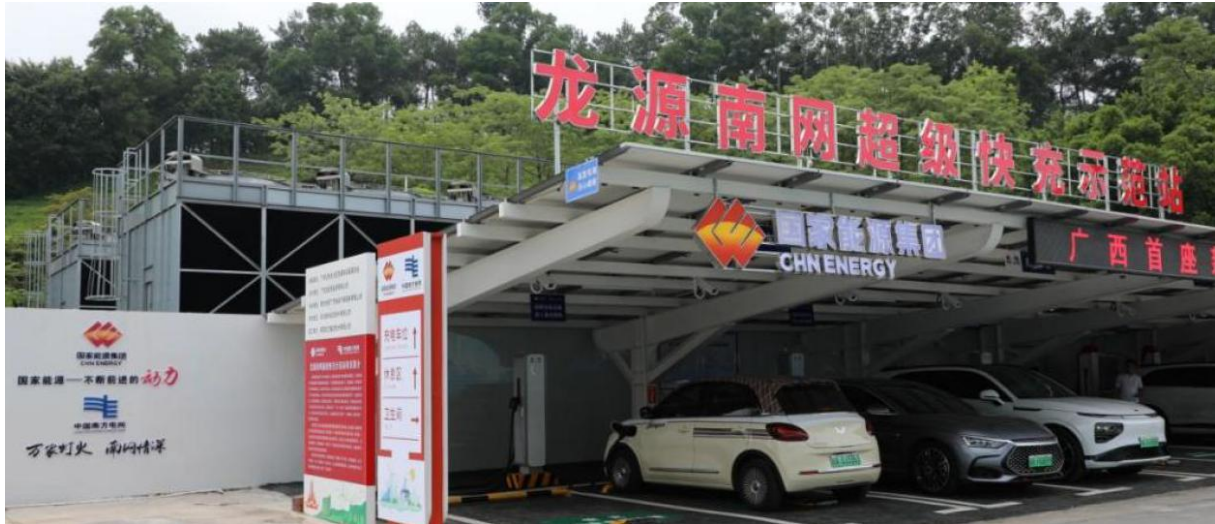
Figure 9-1 Demonstration of Solar PV+storage+EV charging at Guangxi Longyuan Nanning International Convention and Exhibition Center
