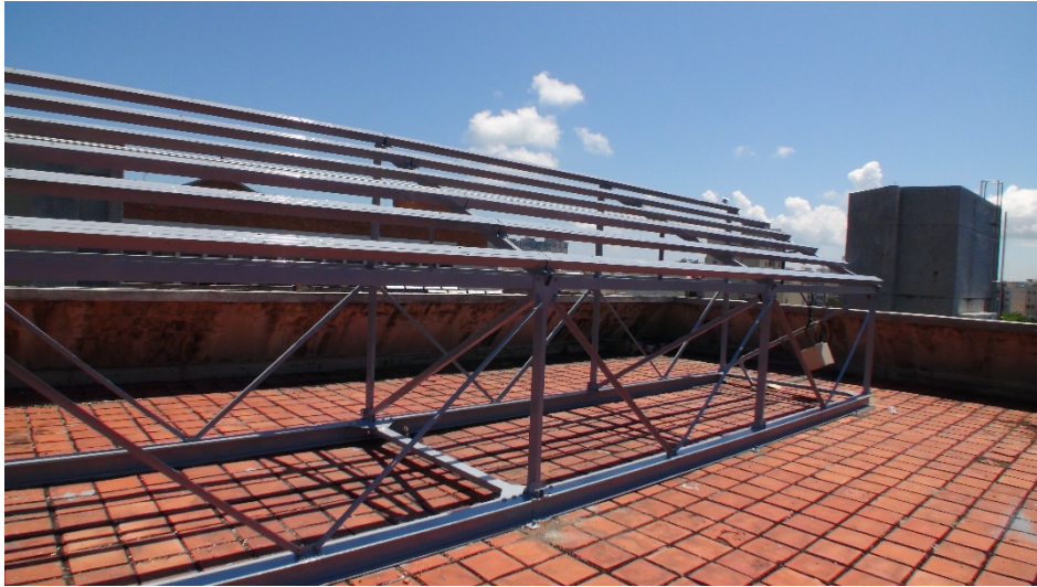
Figure 4.2.5 Finished system bracket
