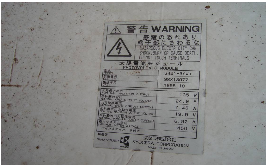
Figure 1.3.2 Module specifications of the Penghu PV system
