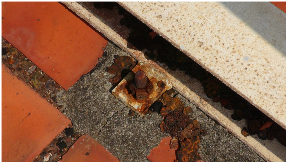
Figure 4.1.6 Status of screws and nuts
