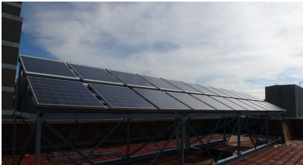
Figure 4.2.6 Modules were installed back to the system bracket
