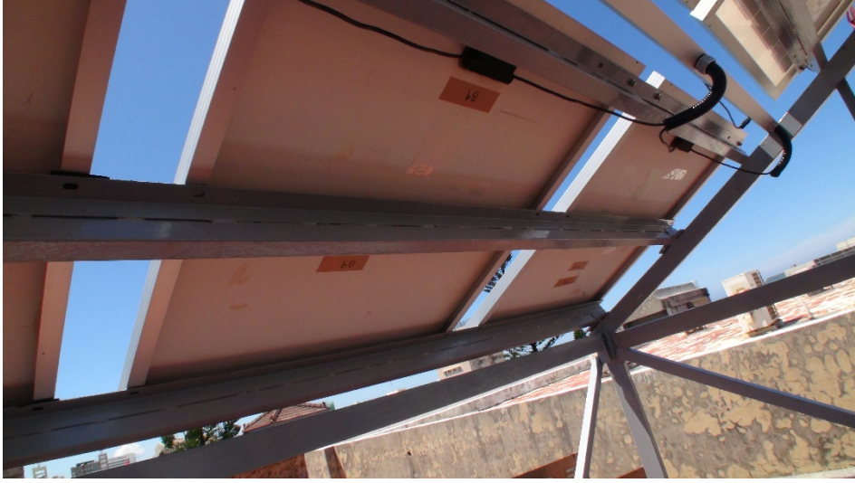
Figure 4.2.7 New DC cable tray
