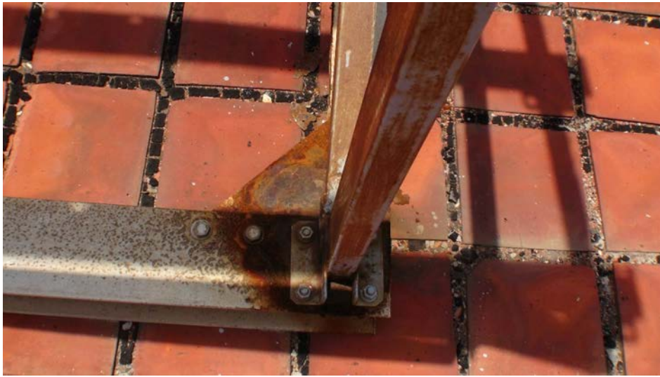
Figure 4.2.1 H shape stainless and the base of bracket after removing rust
