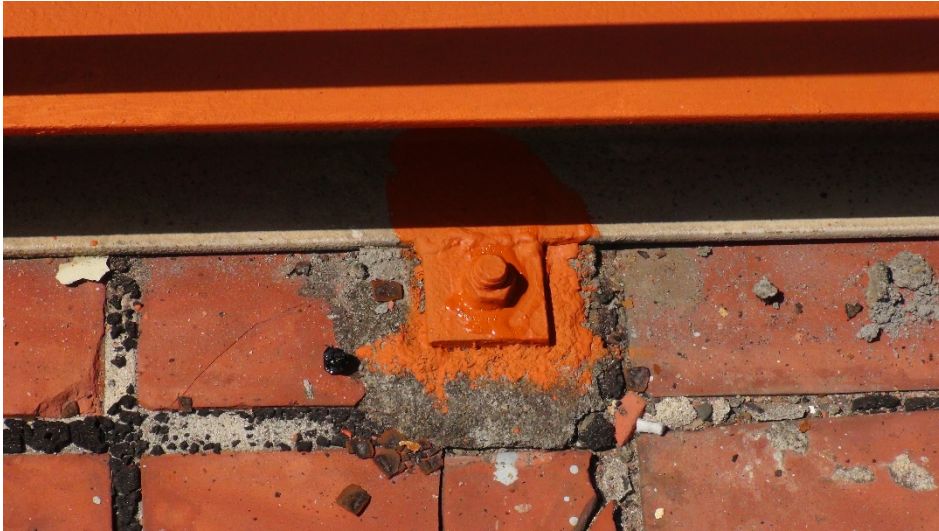
Figure 4.2.3 Bracket base after painting anti-rust paint
