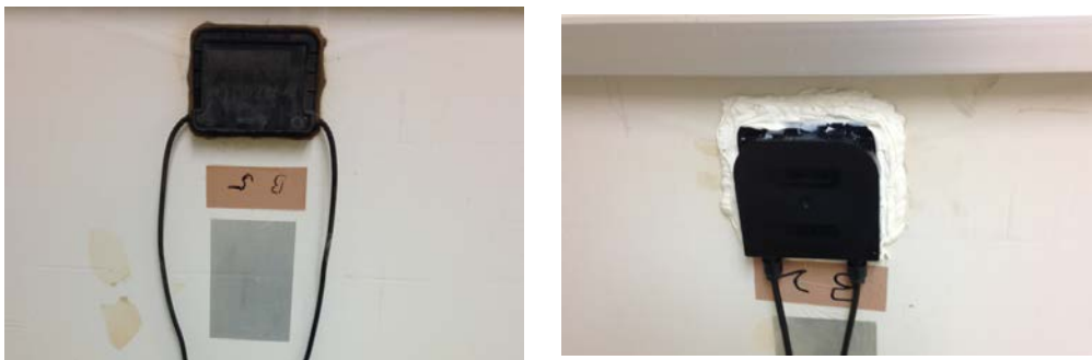
Figure 3.1.2.1 Junction box replacement
