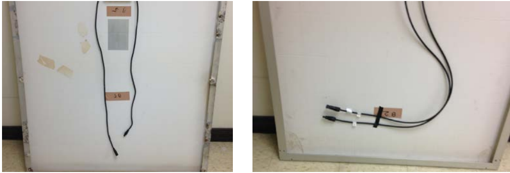
Figure 3.1.2.1 The connector replacement
