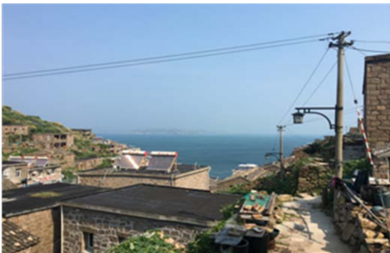
Figure 9 Flat roof of the residence house
