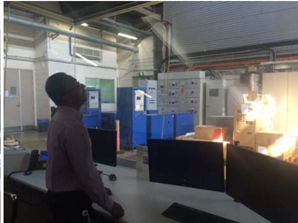
Figure 32 Demonstration of the microgrid
