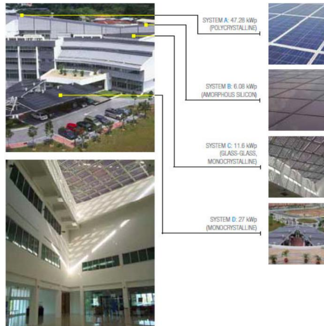
Figure 26: Green Energy Office (GEO) building MGTC
