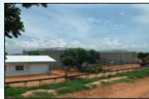
Biogas Project at Northeastern Starch (1987)
