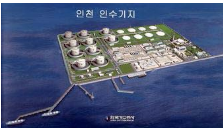
Figure 4.4.2: Model Overview of the Incheon LNG Receiving Terminal (2008) (Source: KOGAS website)
