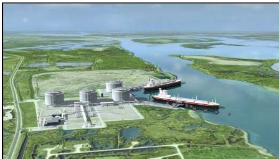
Figure 4.6.2: Cameron LNG Terminal Site Overview (Source: Sempra Website)
