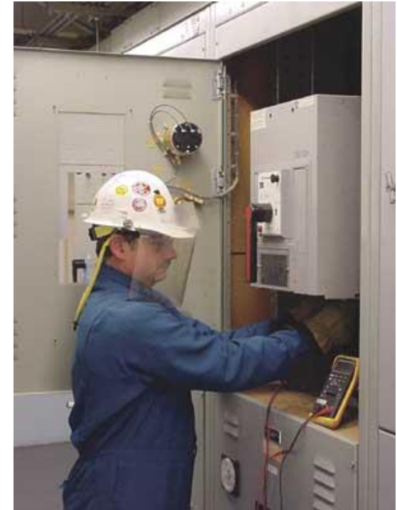
Photo 6. Workman verifying that equipment is de-energized; note protective clothing.
