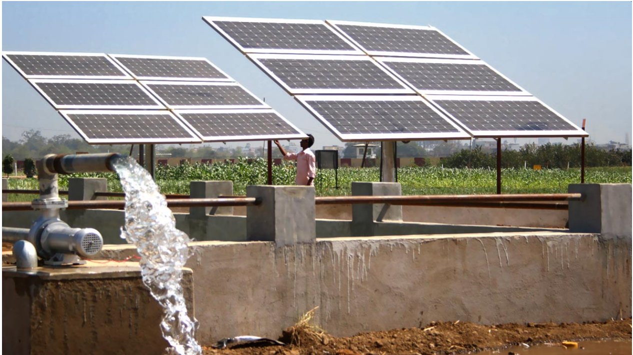
Figure 11. Example of a Solar Water Pumping System
