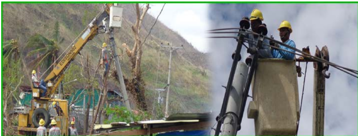
Figure 8. Task Force Kapatid of the Philippines National Electrification Administration at Work
