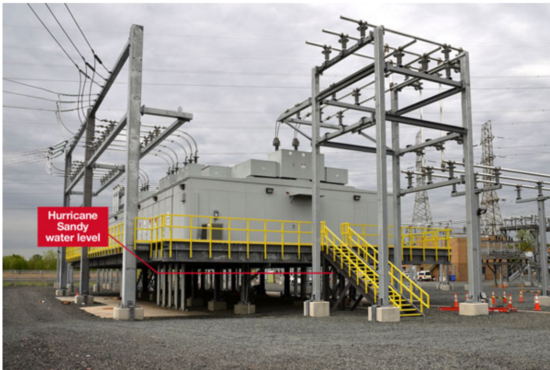
Figure 6. Higher Elevation Design Standard for Substations
