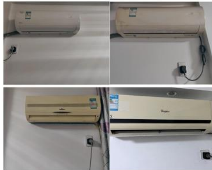
Installation of AC companion
